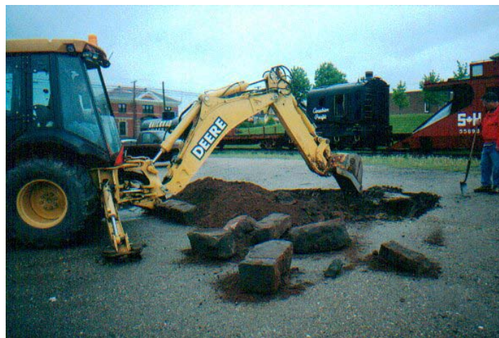
First dig for the station, June 6 2002. Photo by Art Clowes.
